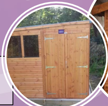
Donation and construction of a new shed for Harmondsworth Allotments.
